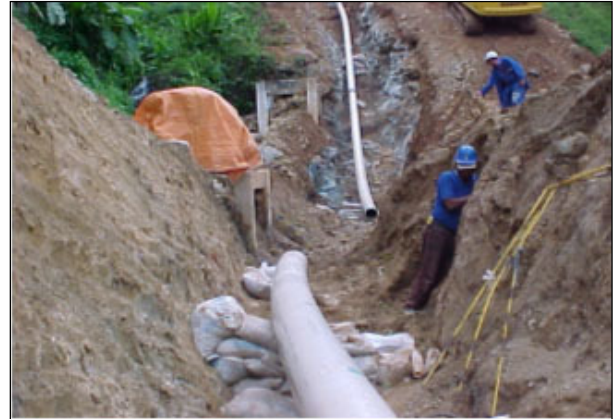
Figure 20: Photo with Pipeline Being Buried
