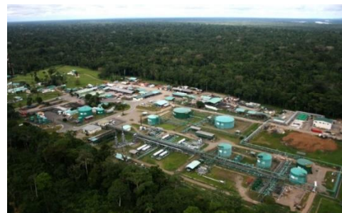
Figure 2. Sansahuari Pumping Station
