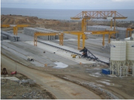
Figure 2: A General View of the Plant during its Construction.
