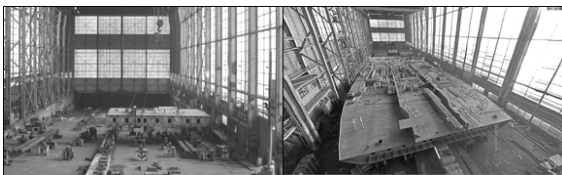
Figure 3: Keel lay event (left) and erected bottom sections during outfitting (right)
