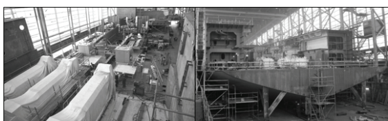
Figure 4: Main engines (left) and big equipment positioned during hull assembly (right)
