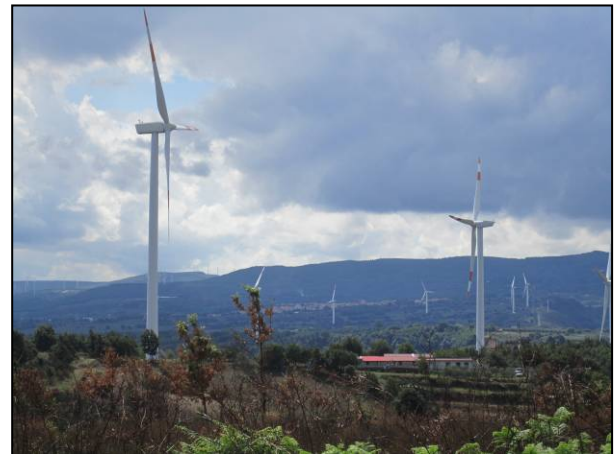
Figure 1: Wind Farm terrain complexity
